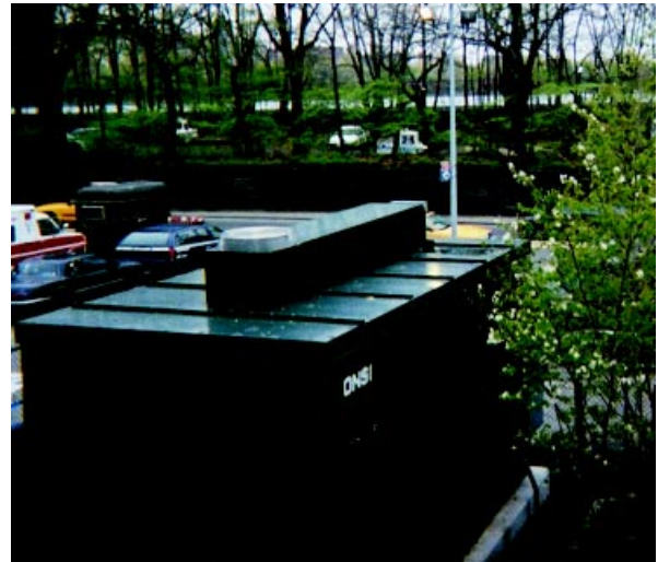
(Left) Early test of small cogeneration featuring a microturbine and absorption chiller on the roof of an Indianapolis drugstore. (Right) Fuel cell in Central Park in New York.
