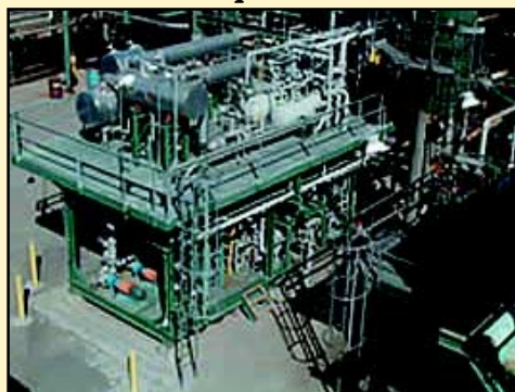
Figure 6: The left photo shows a 260-ton (914 kW) waste-heat-fired absorption refrigeration unit that provides -25^{\circ}\text{C} ( -13^{\circ}\text{F} ) chilling at an oil refinery. The ammonia water air conditioner, shown at right, is designed for microturbine waste heat operation.
